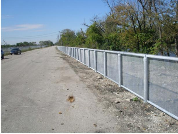
linear feet or 7.48 miles of wire mesh. Their wire mesh product was designed to allow passage of water to relieve flooding but is small enough to block out all but the smallest fish and eggs. This fence project is an environmentally friendly, recyclable solution provided to protect the surrounding natural environment.
